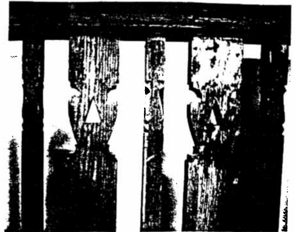
Decorative patterning of the stair balusters was achieved by the simple sawing and notching of flat oak boards which were stained green.
